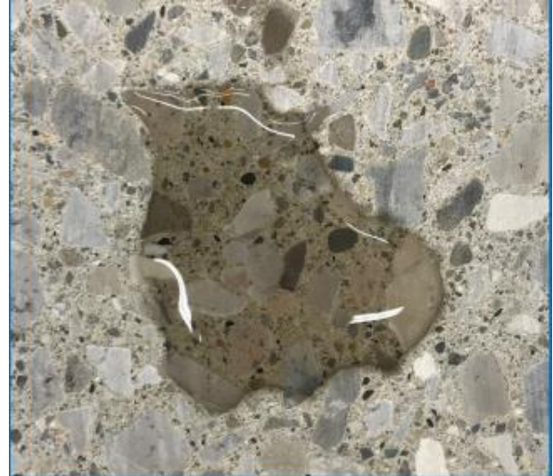
Middle of Treated Concrete
